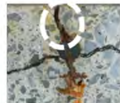
Injected and migrant of corrosion gel through cracks
