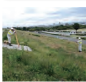
Regular Cross Section Surveying
