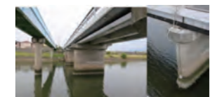
Pilot service in Osaka Prefecture
