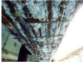
Steel corrosion in concrete structures
