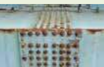
Splice parts and bolts
