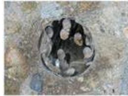
Ducts unfilled with grout
