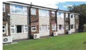
Water heaters as DER in Manchester, UK.
