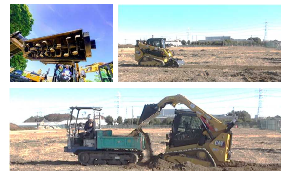
Figure 10: Loosening of the ground using a chiller and soil collection by compact construction robots
