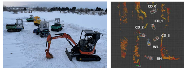
Fig.9 Multiple sensor pods to estimate the location of multiple construction robots.
