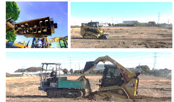
Figure 10: Loosening of the ground using a chiller and soil collection by compact construction robots
