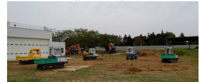
Fig.7 Multi-robots for earth moving operations.
