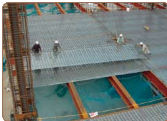
Fab deck floor mold work site
