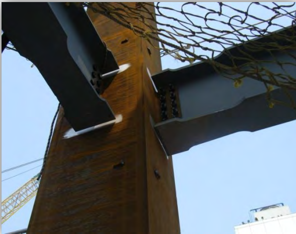
Steel beam-to-column connection
