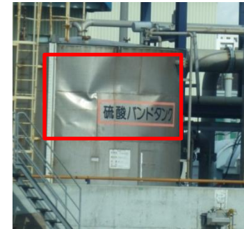
Tanks damaged by debris impact
