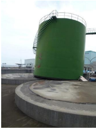
Tank washed away by the Tsunami (Miyagi Pref.)
