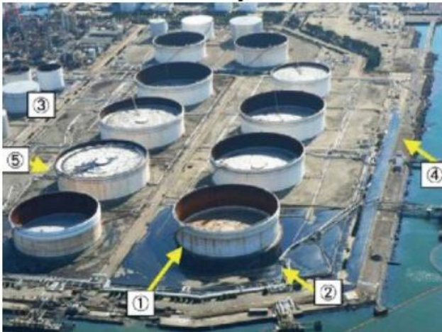
Oil leakage due to collapse of pipelines (Sendai JX Nippon Oil refinery)
