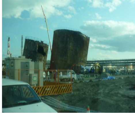
Tank washed away by the Tsunami (Miyagi Pref.)
