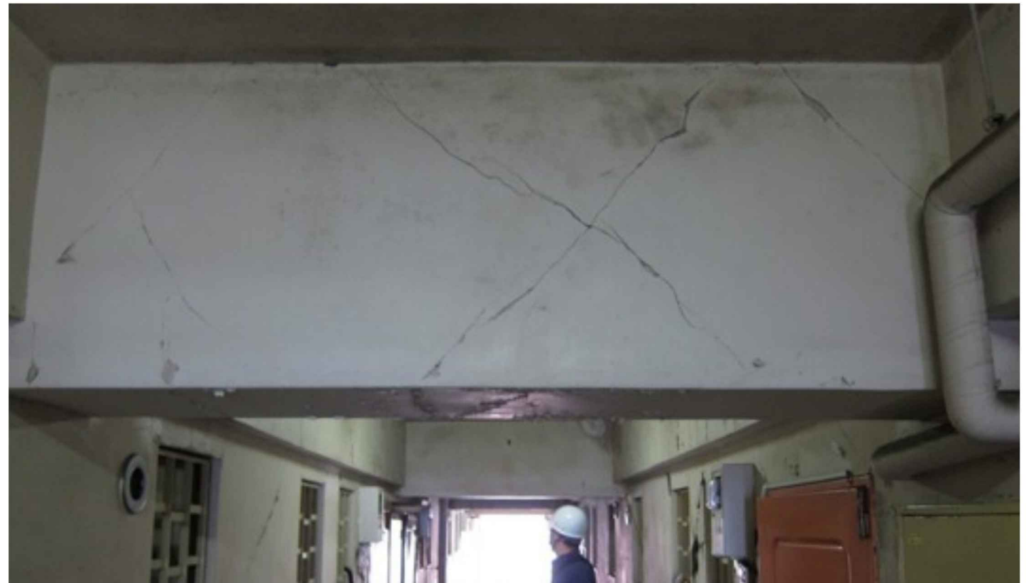
shear cracks on coupling beams
