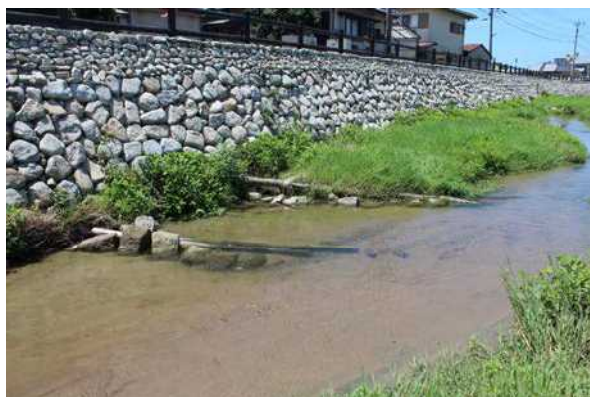
Installed wood structure
