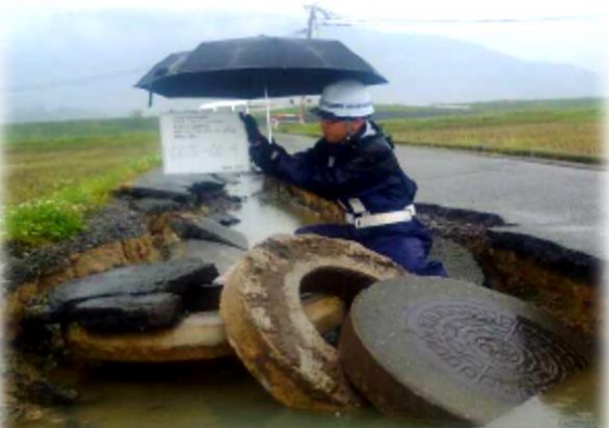
Broken manhole after the earthquake 2)
