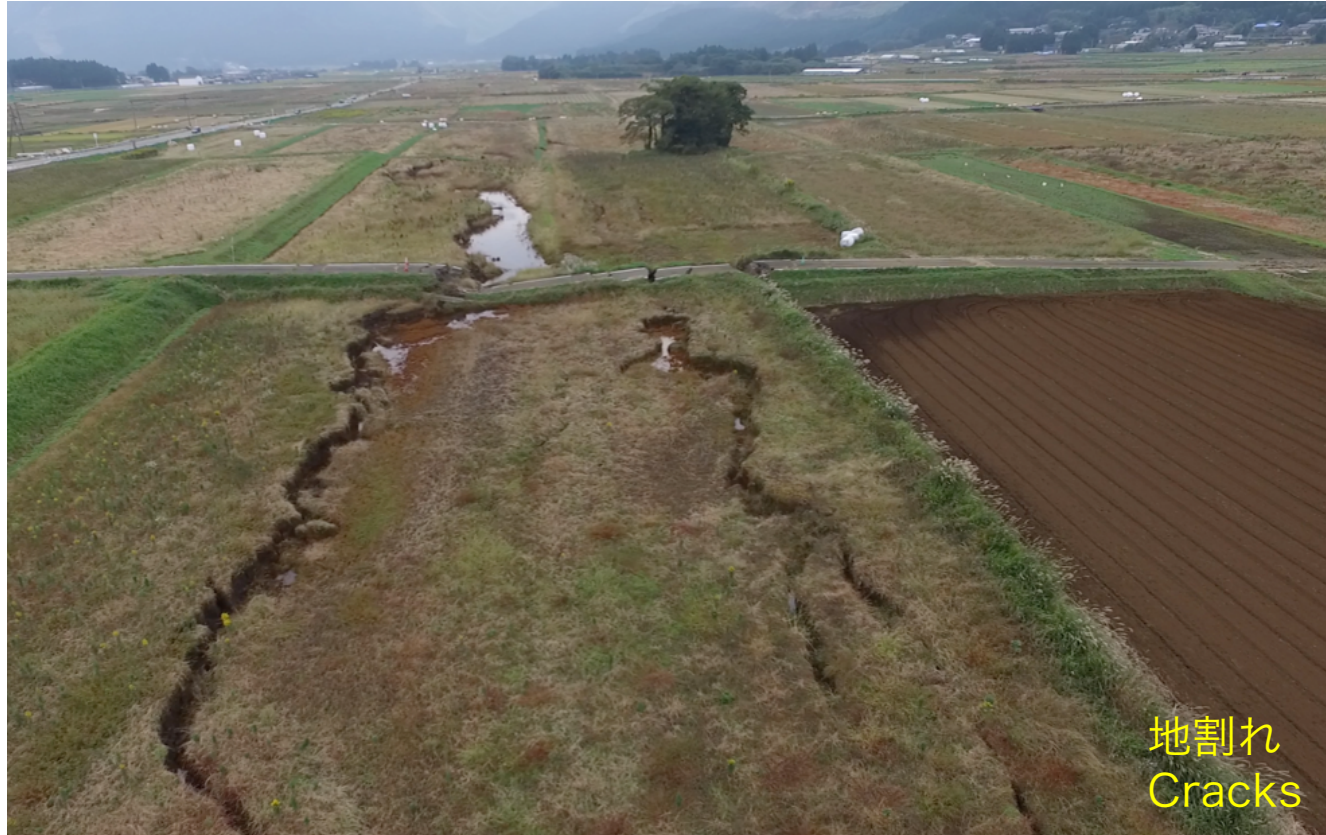
水路の破損 Damage to water channels
