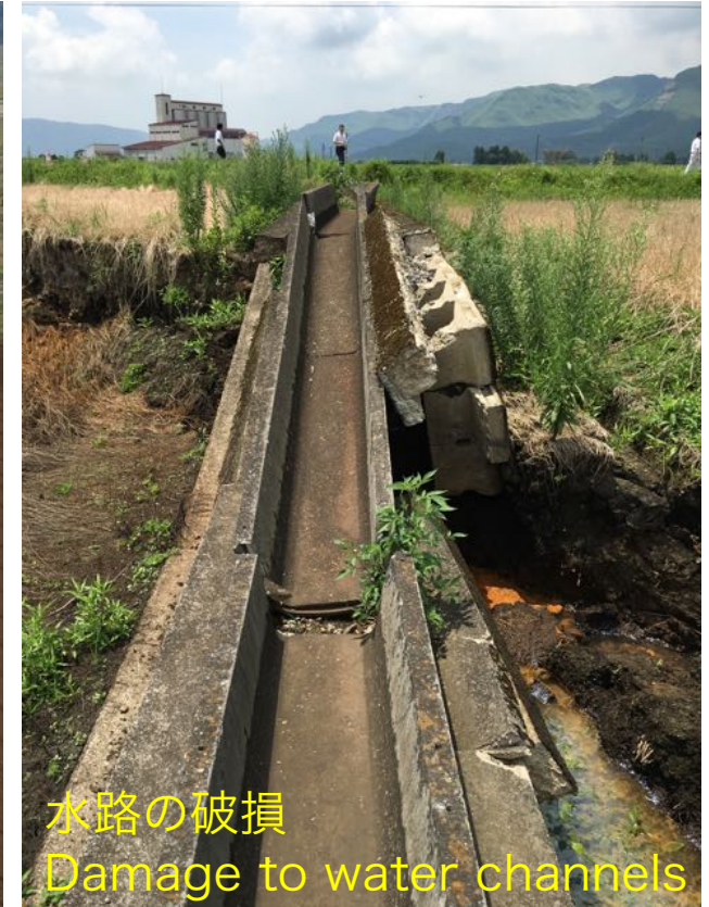
水利施設の人為的破損 Artificial damage to water use facility
