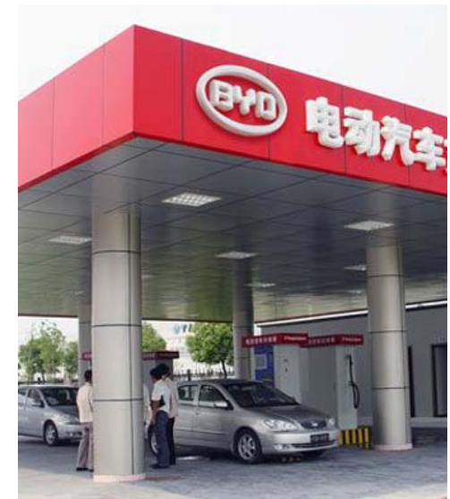
An electricity charge station for EV's in Shenzhen
