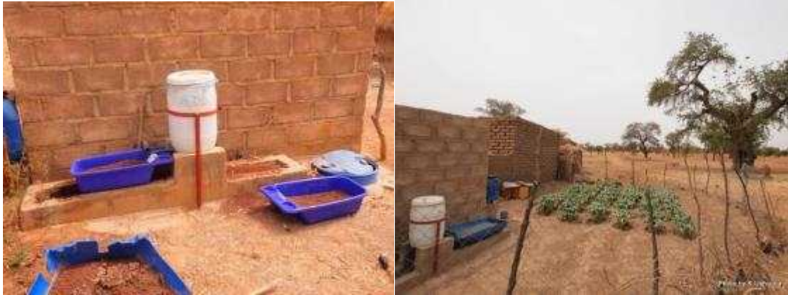
Fig.1 Overview of grey water treatment facility
