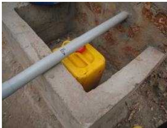
Fig.7 Frame of hole for urine tank
