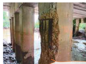
Bridge pier deterioration due to salt exposure
