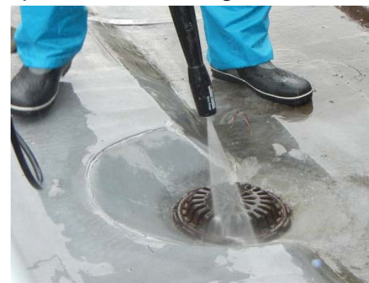
Cleaning by high-pressured water
