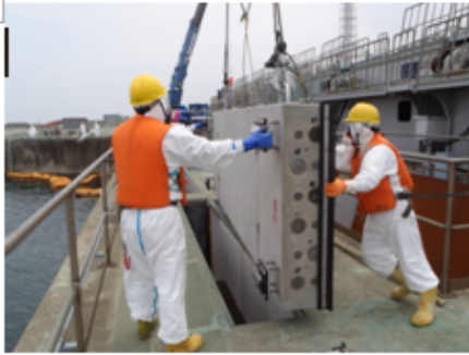
Photograph 1 4 Installation of Stop-Log 4
