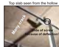
Excessive deformations, cracks of RC culverts have been reported.
