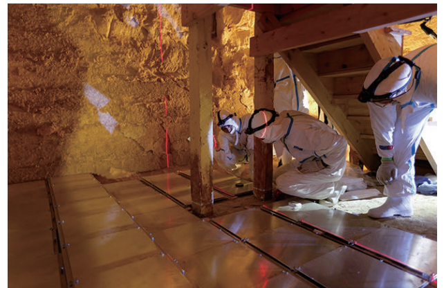
Setting up the nuclear emulsion films within the Bent Pyramid © Scan Pyramids Mission / Ph.Bourseiller
