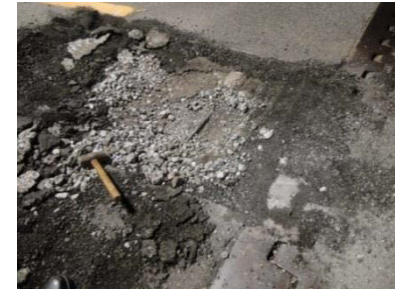
Degradation of concrete slabs
