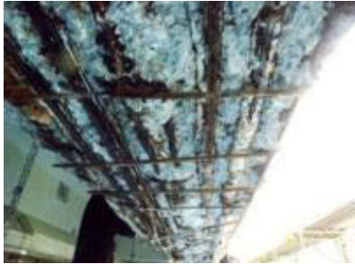
Steel corrosion in concrete structures
