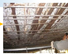
Inner corrosion difficult to find by visual inspection
