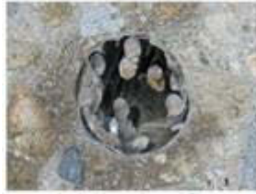
Ducts unfilled with grout
