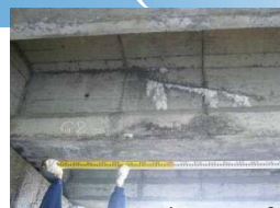
Suspected case of unfilled grout
