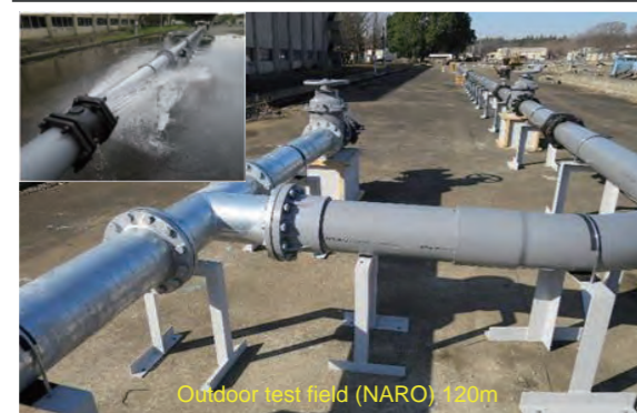
Measurement precision of prototype leak investigation robot now being tested in an outdoor pipeline leak test field. Proving test underway on Miyakojima Island.
