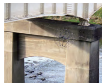
Inspection demo at a real bridge (Chiyoda E. C.)
