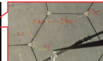
Semi-automatic detection of a crack on a concrete slab
