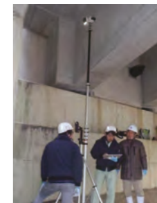
Monitoring of girder end using robotic camera (Elevating Type)
