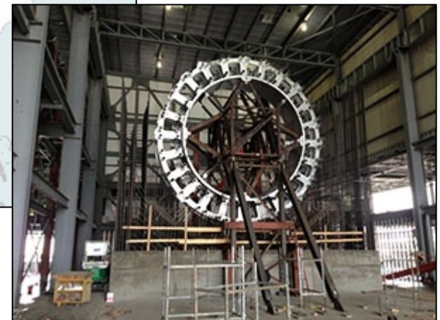
Clemson Drivetrain Testing Facility near Charleston, South Carolina
