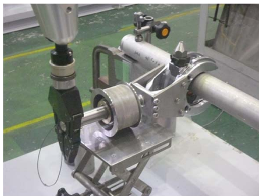
Remote handling cutting and welding of LBE piping for the target vessel replacement
